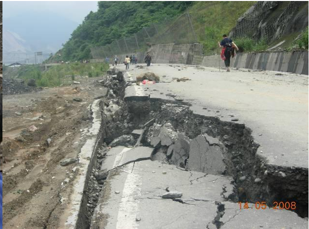
Figure 2: Collapsing of road surface of the highway G213
