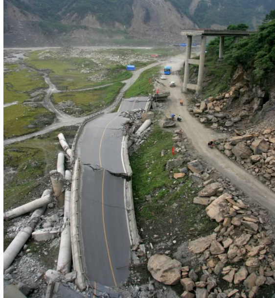
Figure 5: the collapsed Baihua Bridge in the highway G213
