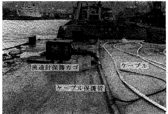
Photo.2 In-site seepage flow meter
