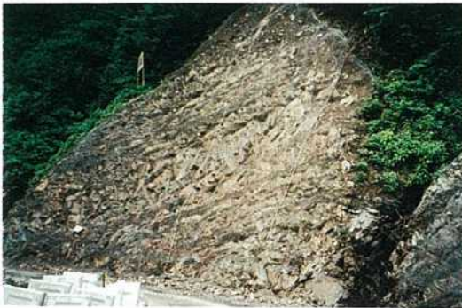
Photo 3 Picture of the excavated slope.
