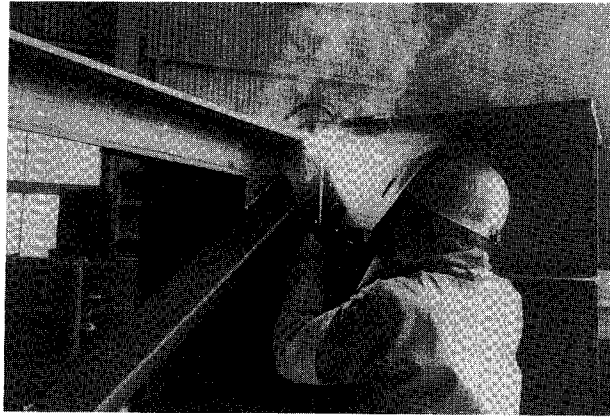
Photo1 Bridge model used for making test specimens.
