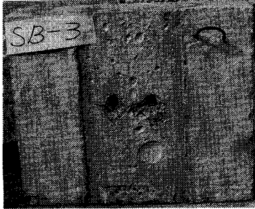
Photo 2 Contact surface between steel and concrete after fatigue failure at (B) Type specimen.
