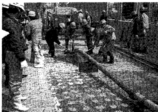
Photo 2 Casting of SFRC.
