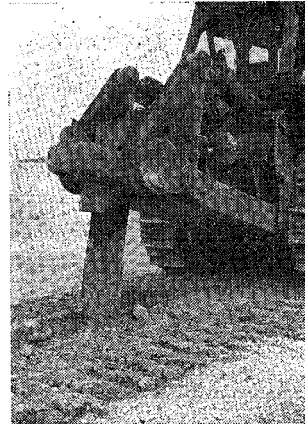
Photo 5 Rippling operation under testing.
