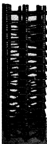
Fig. 3 Reinforcement cage.
