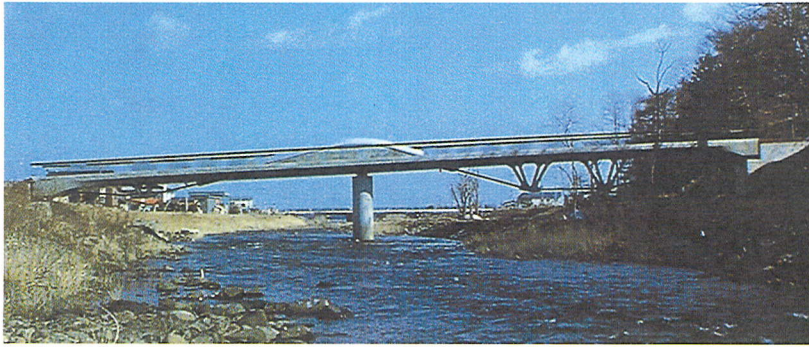
Fig. 12 View of the completed bridge
