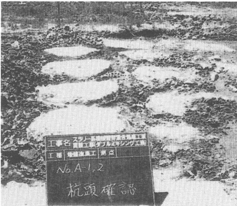
Photo 1 Soil-cement columns after construction
