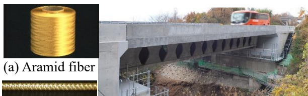
(a) Aramid fiber (b) AFRP rods (c) Opened to traffic since December 2020 Fig. 1 The Bessodani Bridge
