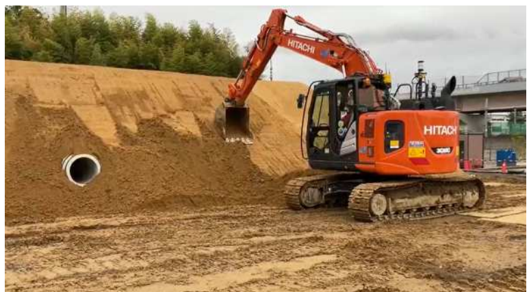
図-6 ICT 建機法面整形
