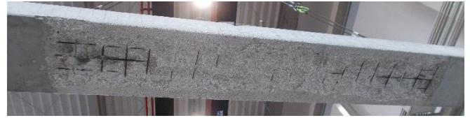
Figure-3 Explosion Spalling condition after heat test
