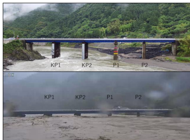
Fig.2 Bridge during normal river water and swollen river water.
