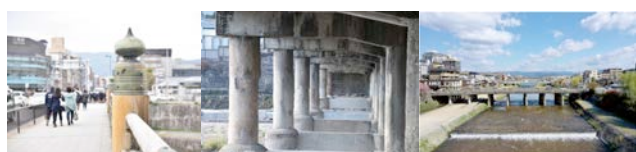
(a)擬宝珠付き木製高欄 (b)石柱橋脚 (c)多柱式構造
