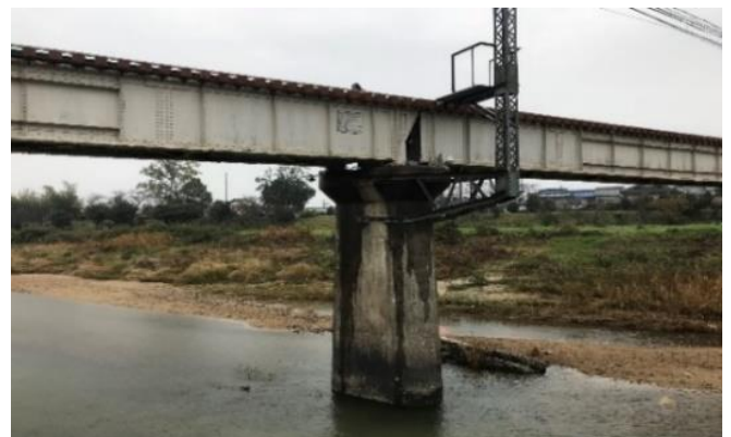
Fig.1 Photo of target pier.
