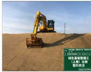
写真-3 ICT 建機法面整形工
