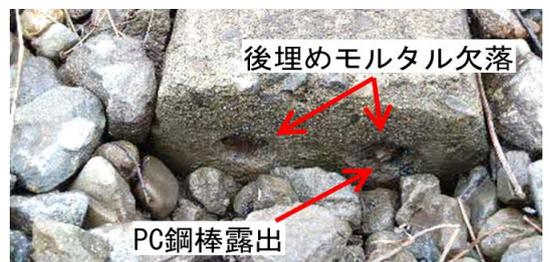
図-7 PC 鋼棒露出
