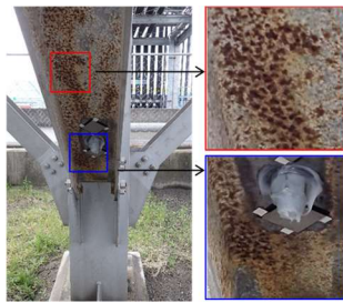
Fig.1 Structural trusses with hot-dip Al coating in a trestle bridge after service for 25 years.
