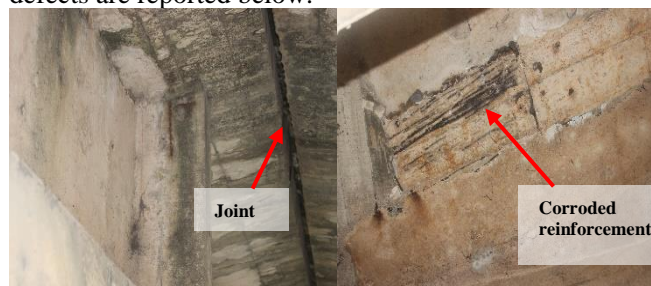
Fig.3.Corrosion of reinforcement in slab and column
