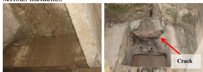
Fig.4. Spalling at the connection of slab and wall column
