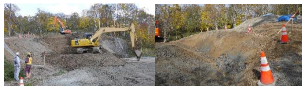
Photo.2 Construction yard foreground (left), excavation slope (right)
