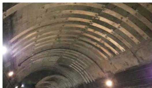
図-2 帯鋼板の施工例<sup>2)</sup>
