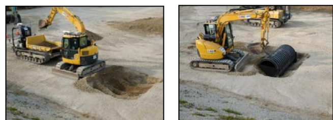
(a) 掘削・積込
