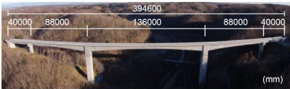
Photo 1 View of Obirashike-river bridge.
