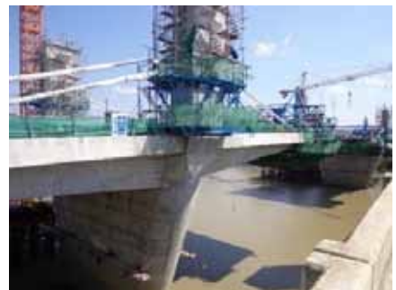
Fig.8 Construction of PC Extradosed Bridge
