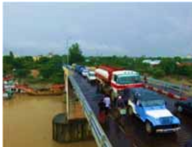
Fig.2 Existing Thaketa Bridge
