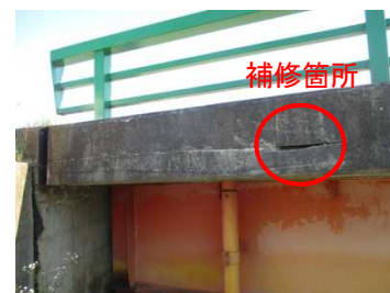
図-3 補修実証橋梁
