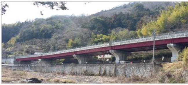
Figure 1: Sanbonmatus bridge overview.
