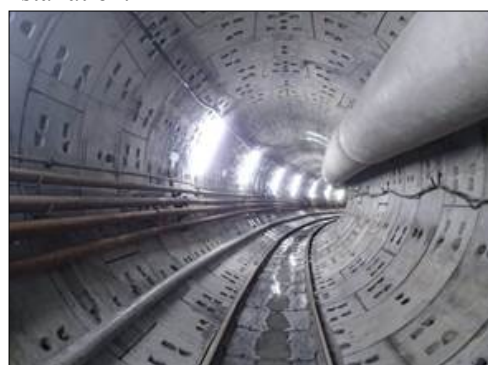
Figure 5 RC Segment Lining during Construction
