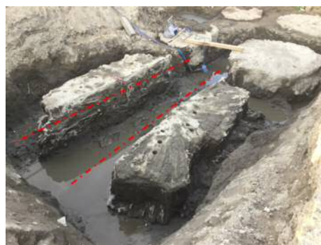
図-6 矩形改良体掘り出し後(全景)
