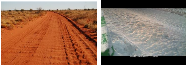
Figure 1 Left: Washboarding on dirt road (Photo by Leprechaun, The Navara Forum). Right: Snow corrugation (Photo taken at Hokkaido University)
