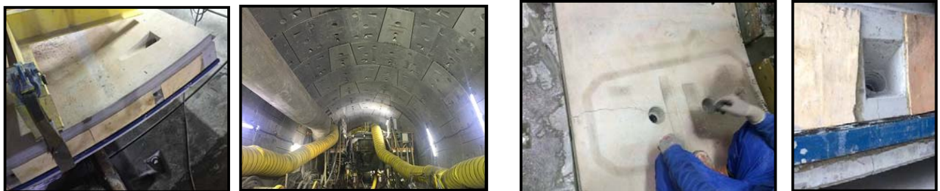
Fig 3 Gasket/Plywood and Segment inside Tunnel
