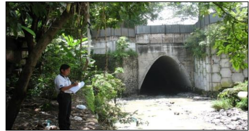
Fig.2 Narrowing of Channel limiting Hydraulic capacity.
