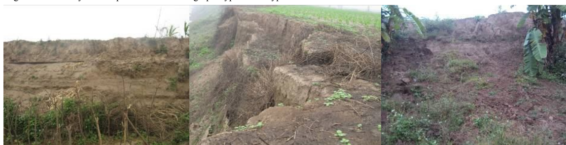
Figure 4. Failure river bank (pictures took in Ngoc Thuy, Xuan Canh, Hai Boi)
