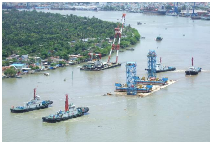
Photo.1 Towing of Tunnel Unit
