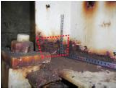
Photo 1. Stiffener damage in corroded plate girder (Tamakoshi, 2006)
