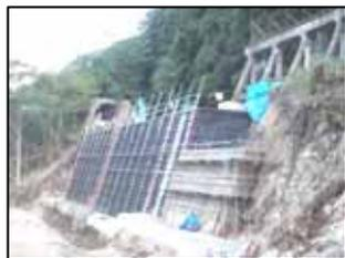
写真-5 盛土補強土壁構築
