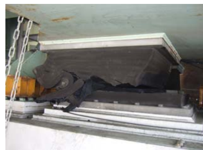
写真-1 P52 支承
