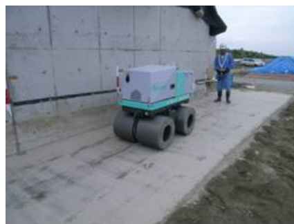
(c)難透水性覆土転圧
