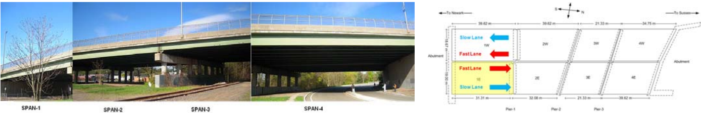
Figure 1. View and layout of tested bridge
