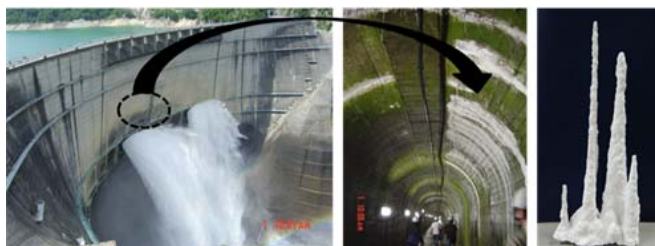
Fig. 1 Formation areas of secondary phases in the inner tunnel of Kurobe dam (Japan)
