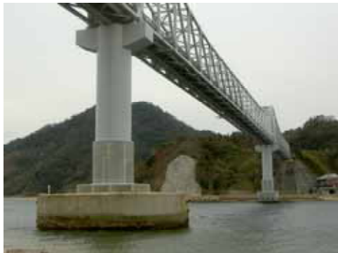
(a) P1 橋脚側
