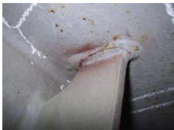
図-1 縦桁補剛材天端のき裂
