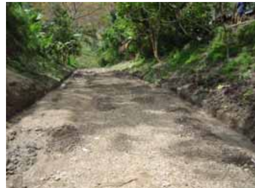
Photo.4 The road after the construction
