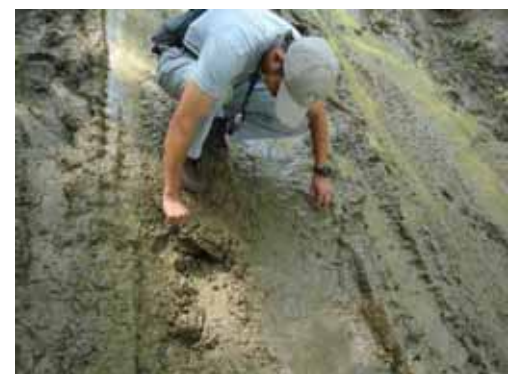
Photo.5 The road 3 months after the construction
