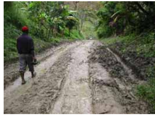
Photo.3 The road before the construction
