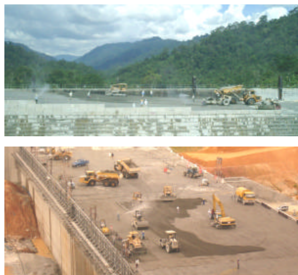
Fig- 2 Spreading and compacting RCC by SLM
