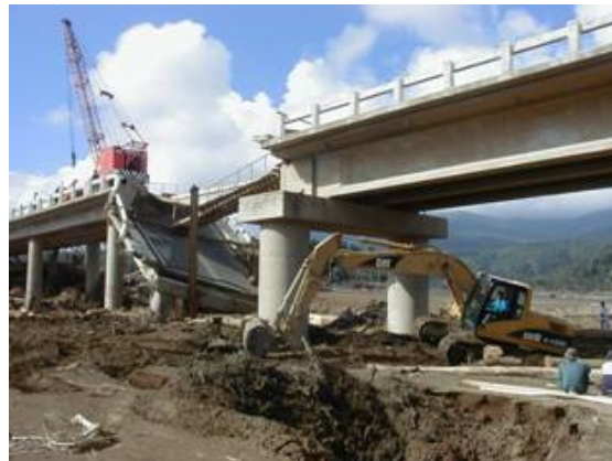
Fig. 3. One of the bridges washed-out by debris-loaded floodwater.
