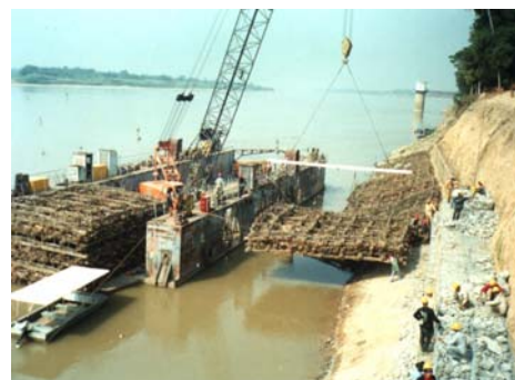
Fig.3 Installation of Fascine Mattress
