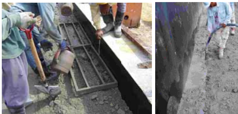
Fig-4 Pouring and vibrating GE-RCC
