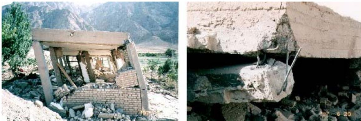
**Fig. 1** A typical R/C building (Ardakul) suffered by joint failure and slip out of plain bars
