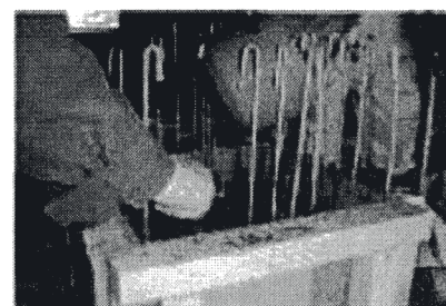
Fig 1(b) Spacer rods between Mesh Layers
