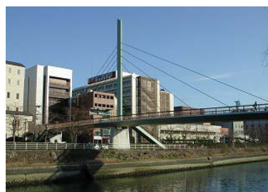
図-6 計測対象橋梁
